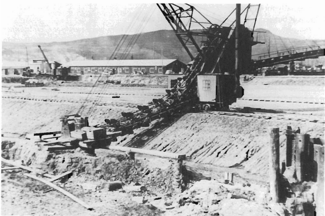
Putting in wall footings for Dora I. Some of the shuttering for keeping the site dry can be seen in the foreground.
