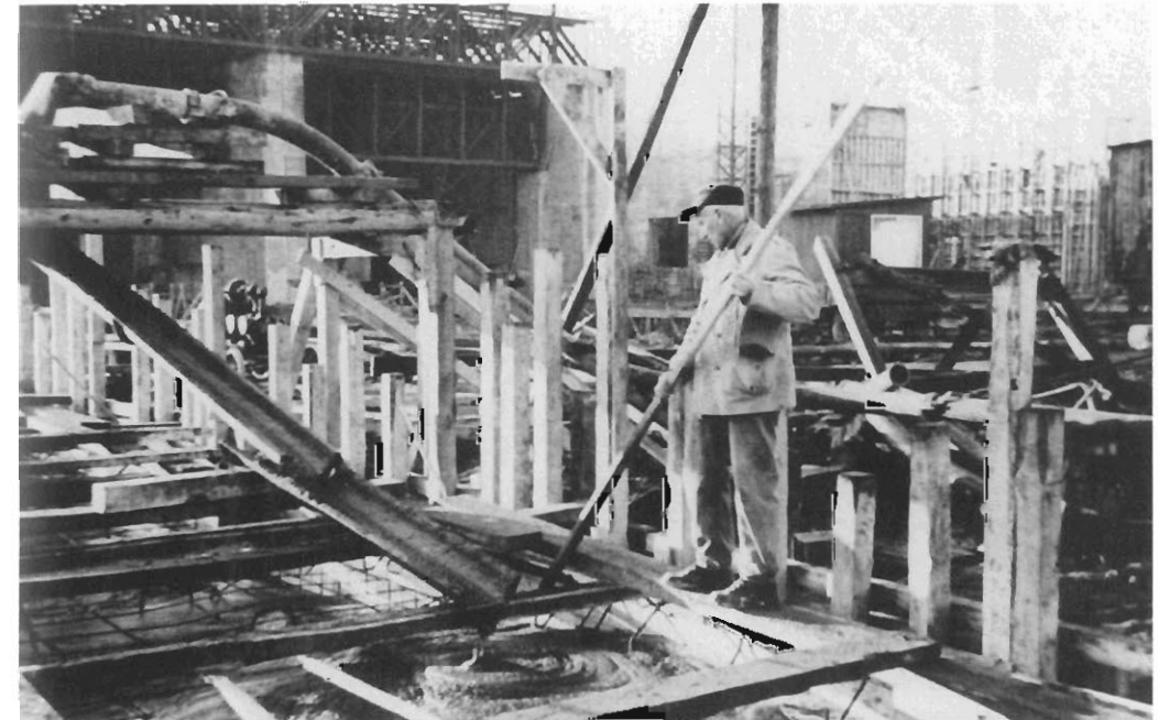
The making of Dora I in Trondheim, with part of the roof being put in place in the background. Once the walls were high and firm enough, it was possible to put the roof girders in place. Most of the metal visible in the distance was later covered with wooden shuttering to be hidden inside the solid, thick roof.
