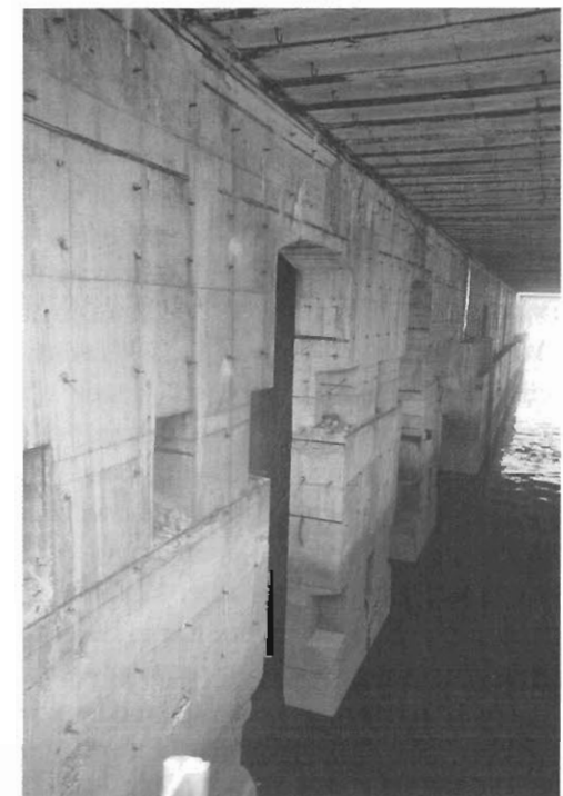
The inside of the Hornisse bunker in Bremen showing the centre wall and the low water level of the river Weser. This is tidal and the dark green algae of the high water mark can be made out against the lighter coloured concrete. The walls look rather thin, but there were two of them, side by side with a narrow gap in between.
