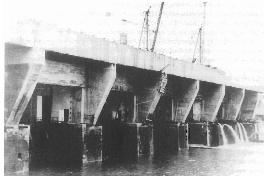
A close-up of the narrow single, dry pens at Brest, with water being pumped out of those towards the right. The drainage gear for these was one of the early weak points, being rather slow at emptying the huge basins. This problem was later overcome by fitting a channelling system so that a number of pumps could be connected to any combination of pens.
