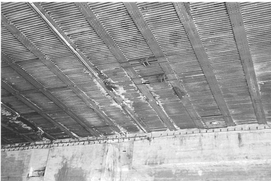
The ceiling of the lock bunker at La Pallice. There is very little to see because the majority of the steel beams have vanished into the concrete and all that is left down below are the bottom edges of the beams and the corrugated iron shuttering which held the near-liquid concrete in place.
