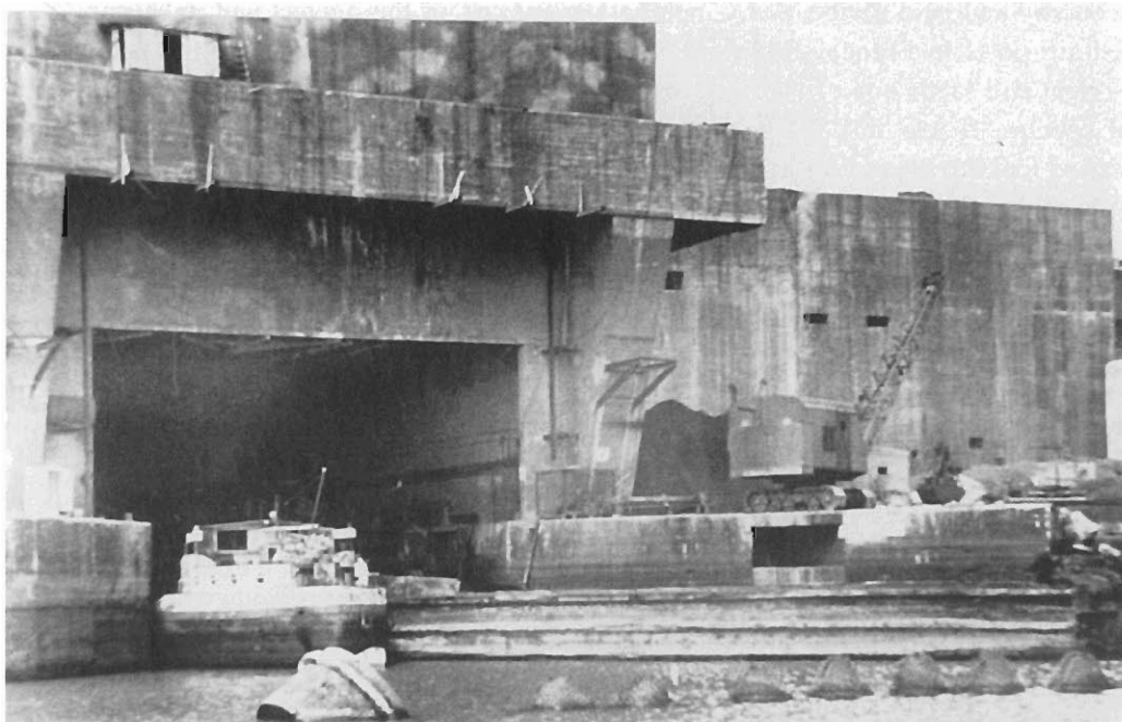
A close up of the single water entrance of Keroman I. This huge gateway was situated on the left hand side of the bunker as one looks at it from the sea and the main body of the building stretched away towards the right. In the foreground are the floats of a torpedo net.
