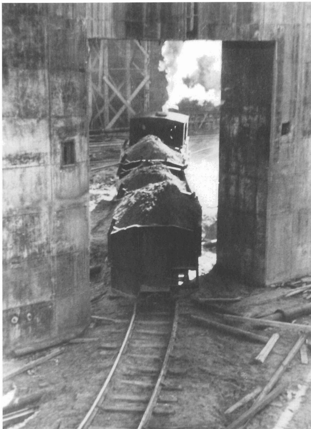
Sand and gravel being delivered to cement mixers inside the large Valentin bunker at Farge near Bremen. Mixers were accommodated in sheds by the side of the bunker so that the wet concrete could be pumped to where it was required, but this was not always possible and highly precarious road and rail systems were constructed to bring in vital supplies.
