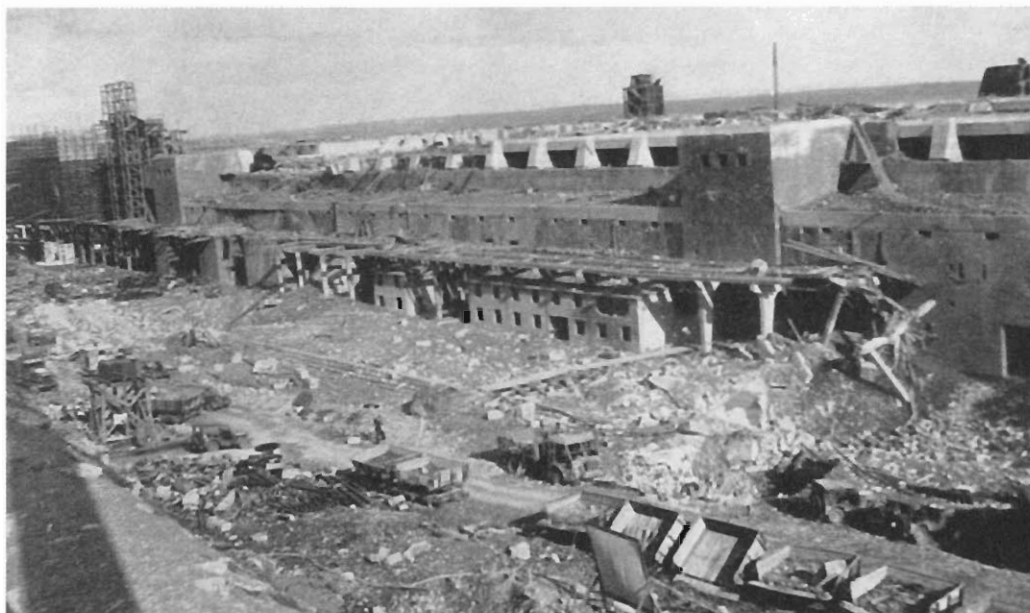
Below: The rear of Brest bunker with extensive bomb damage, but with the concrete apparently untouched.
