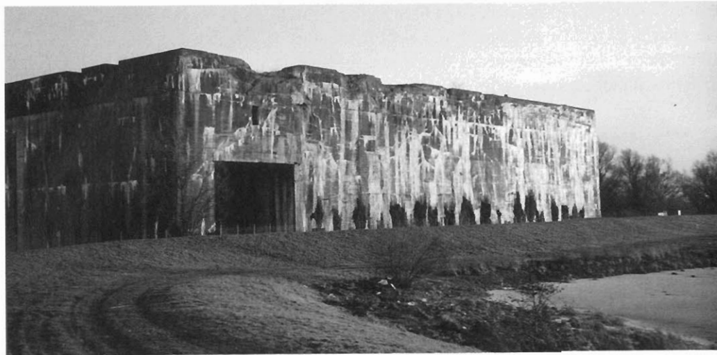
Although the Valentin bunker is almost half a kilometre long, it is not terribly wide, as can be seen here on what was the river or exit side of the production line for Type XXI U-boats. Much of the building has been hidden behind a thick layer of trees. The damage to the roof was done after the war when the bunker was used as a target for bombing trials.
