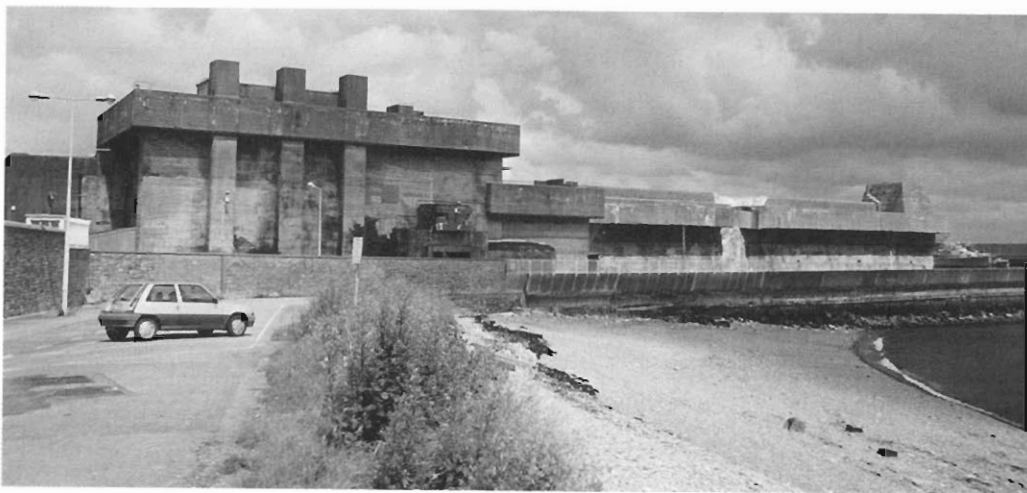
The west side of the Brest bunker with the entrance to the right of the three pillar-like supports running up to the high section of the roof. Bomb damage from a Tallboy striking the edge of the roof can be seen about halfway along the lower section of the roof. There is an anti-aircraft emplacement for a small calibre gun on top of the roof at the extreme right-hand corner.
