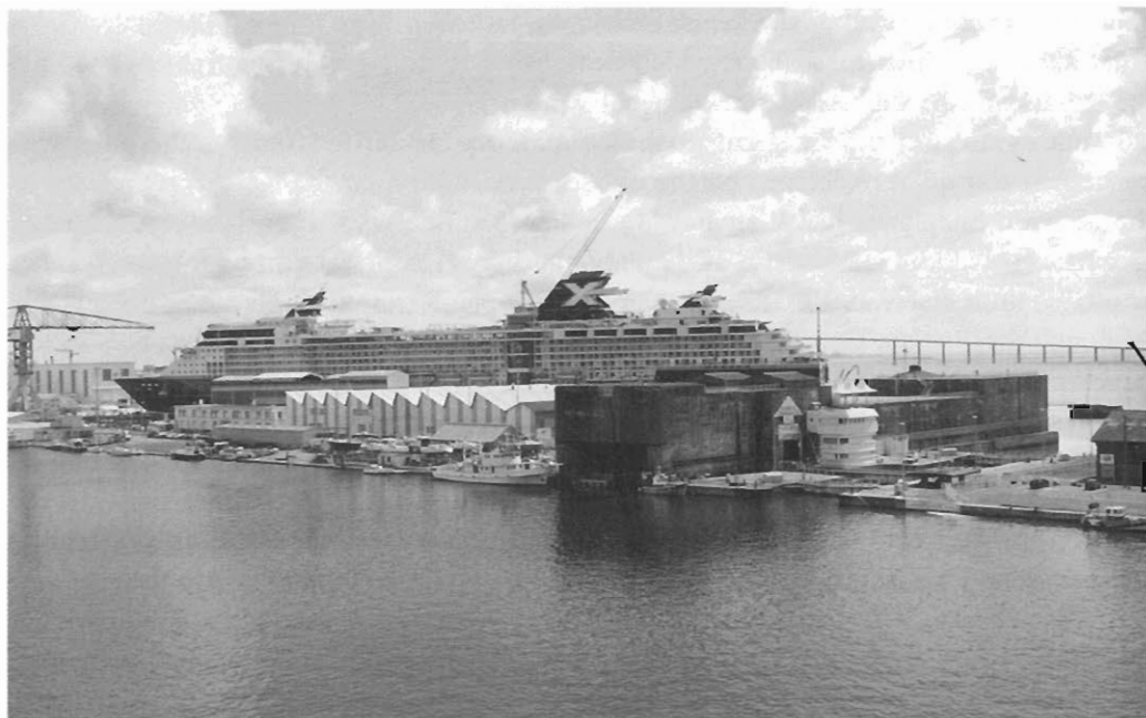
Looking down at the Brest bunker from a road running up the old sea cliffs behind it. A modern white screen has been put up along the top edge of the roof, but the white supports for the dark grey beams of the bomb-catching grid can be seen. Sticking up, towards the left of the picture is a tower left over from the wartime anti-aircraft defences. The two small, shed-like roofs are of special interest. These cover the holes made by Barnes Wallis's bombs and prevent rainwater from washing into the pens below.
