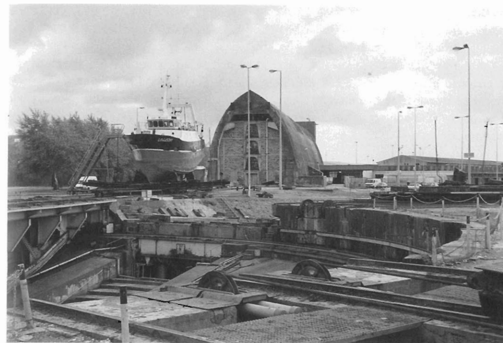
The Eastern Dombunker and massive turntable with one of the many-wheeled buggies for carrying ships onto dry land.
