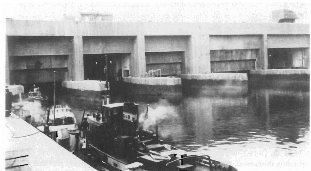
Dora I in Trondheim showing the heavy portcullis type of armoured doors. Sliding down from the ceiling, these could shut off the space between the roof and water to prevent pressure waves from bursting bombs shattering the inside of the bunker.
