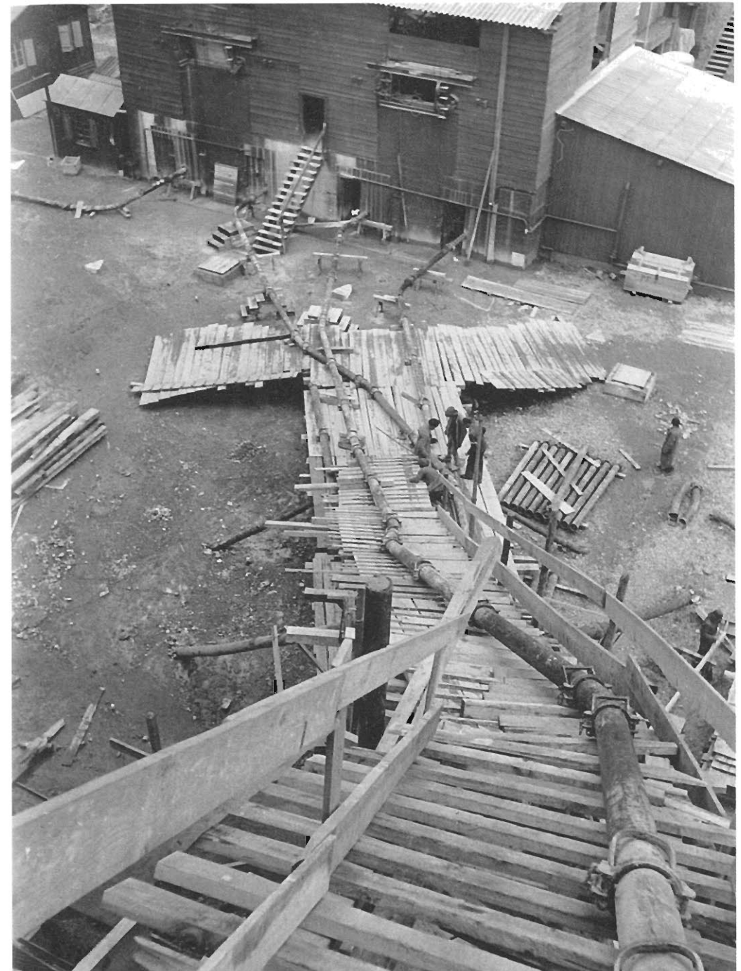
Peering down the so-called 'ladder to heaven' from the roof of the bunker at Bordeaux. Although rickety looking, these structures had to carry considerable weight and be wide enough for a good number of men to undo the joints when the pipes clogged. The building in the background housed both cement mixers and pumps. Bad weather was a special problem during northern winters, when there was a tendency for water to freeze in the pipes.
