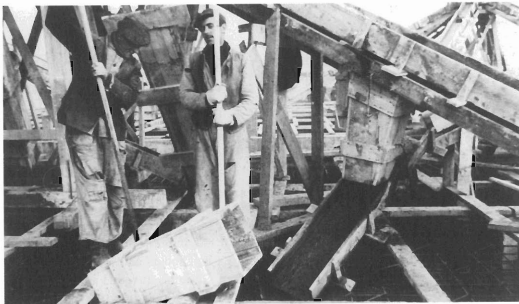
A close up of the cement being agitated while it settled into its mould. Seeing this, one immediately wonders how many men actually lost their concentration to fall into the slushy mix. Working high up, on cold and exposed timbers of the U-boat bunkers must have demanded not only a great deal of determination but also considerable physical and mental effort.
