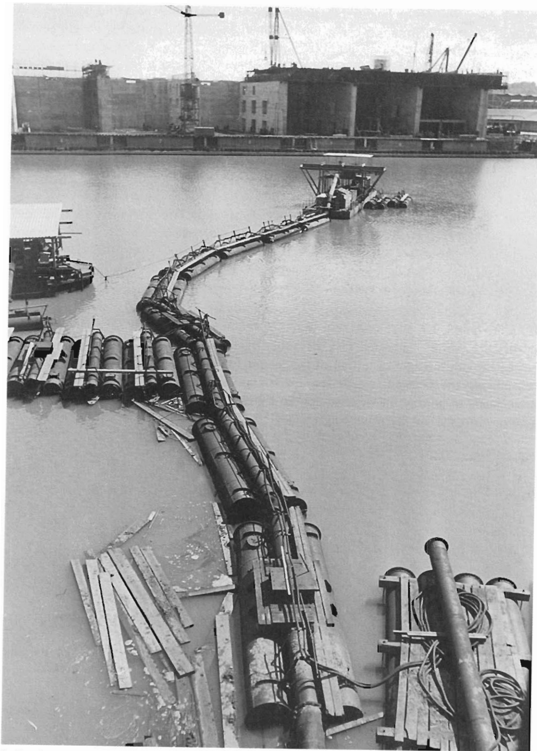
In Bordeaux, space was severely limited for accommodating the vast machinery needed to build the bunker and some of the cement mixers were such a long way away that the pipes had to be floated over the port basin on makeshift rafts, as can be seen in this picture.
