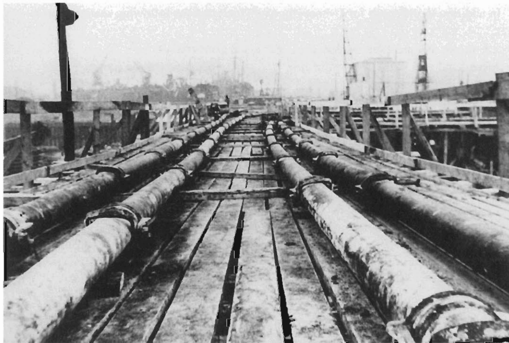
The wooden shuttering of the Dora bunker in Trondheim carrying pipes from the cement pumps. These worked relatively well, as long as there were no great air locks nor any solid lumps in the system.
