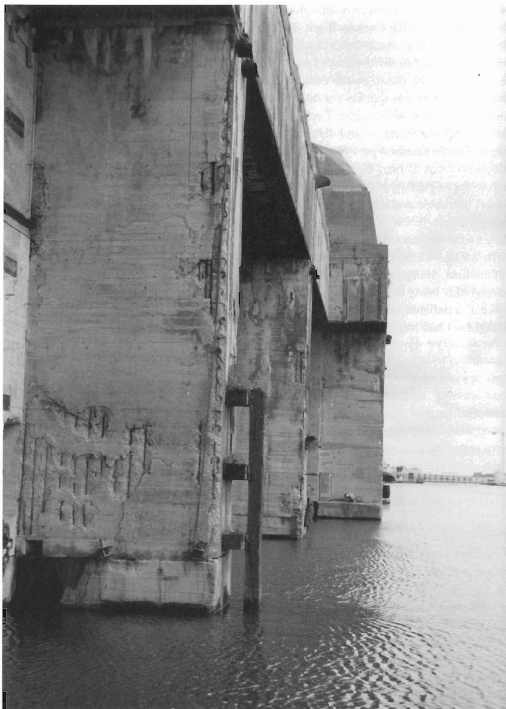
The massive dimensions of the U-boat bunkers are best appreciated by standing close to them and peering up at the overpoweringly thick concrete beams. This shows the water side of the bunker at St Nazaire with an anti-aircraft battery protruding above the wall in the far distance.
