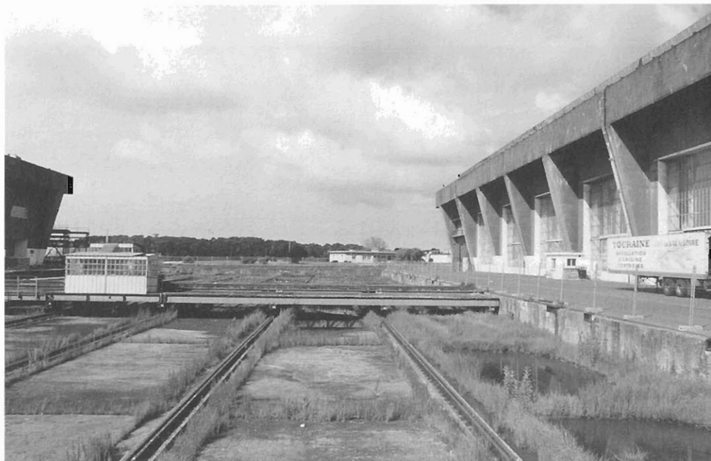
The eight-rail wagon for sliding buggies with U-boats in and out of the two bunkers, Keroman I towards the left and Keroman II on the right. The low armoured doors of the buggy bay are still visible in the far distance on the right. The other armoured doors have been replaced by glass partitions to let in light so that the bunker can be used for commercial purposes.
