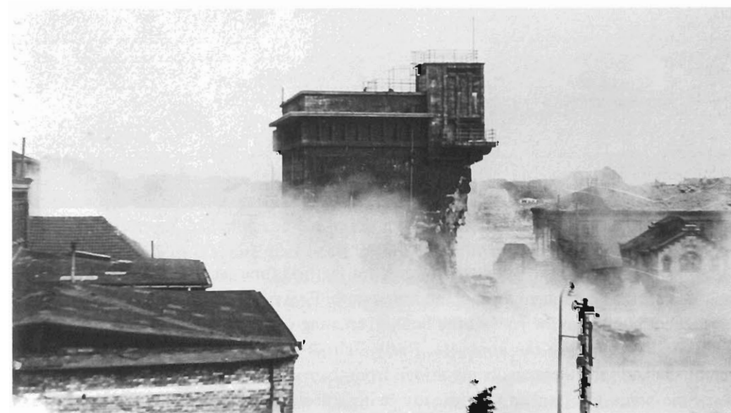
One of the command bunkers in Wilhelmshaven during demolition. Some of this was quite intricate work and even old torpedo nets were hung over bunkers to protect windows in nearby buildings from flying concrete.
